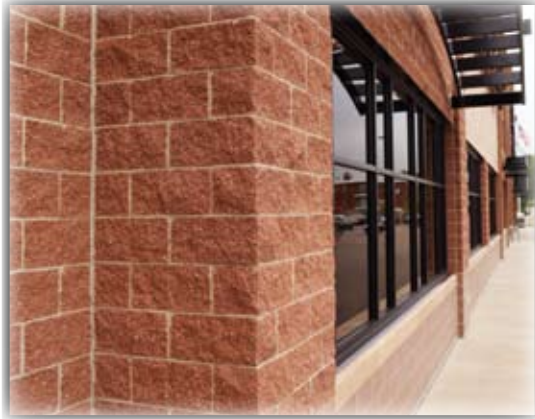
Concrete Masonry Unit with Rockface Finish
