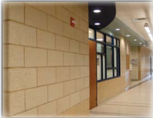
Concrete Masonry Unit with Burnished Finish
